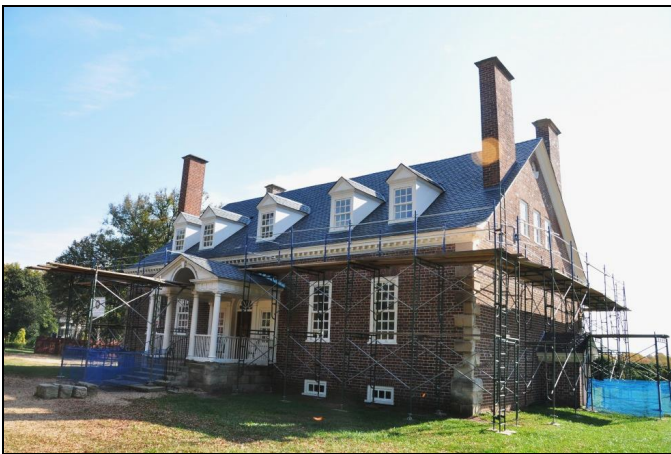
Gunston Hall (Renovation in Progress)
