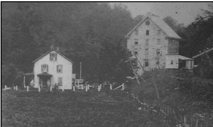
Late 19 th century house by mill
