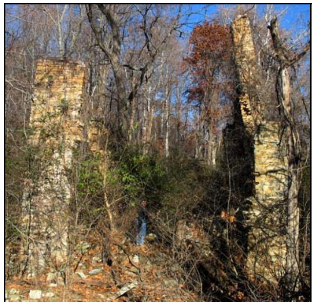
Wall remnants of the old stone Chapman House
