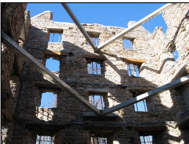
Interior mill walls
